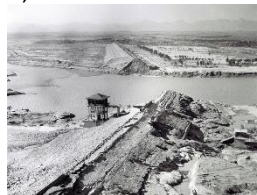
Banqiao dam failure; China, 1975
