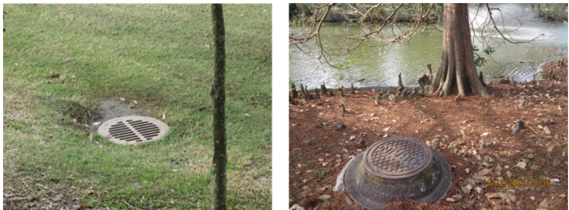
Figure 3.8: Storm drainage in Audubon Park is discharged into urban storm drainage subsystem (and not into ponds).
