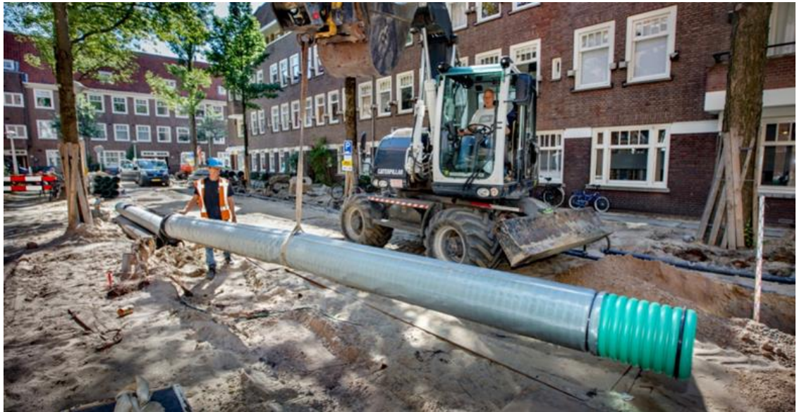
Figure 5.5: Installation IT-drain in Amsterdam (Amsterdam Rainproof)
