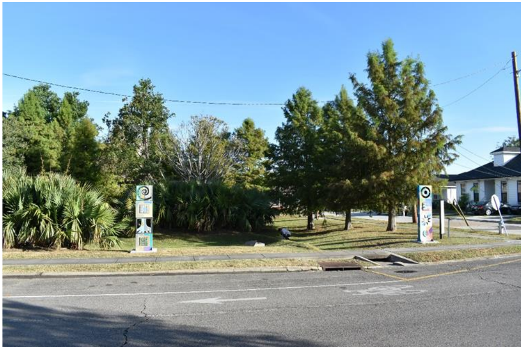
Figure 2.2: example of green infrastructure in New Orleans: test location 2 with signs on the right of the inlet. https://www.climatescan.nl/projects/7399/detail .
