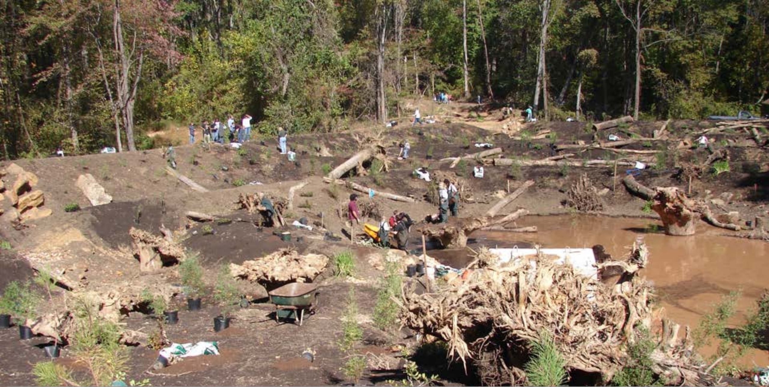
Floodplain reconnection and natural flood attenuation, Washington, DC
