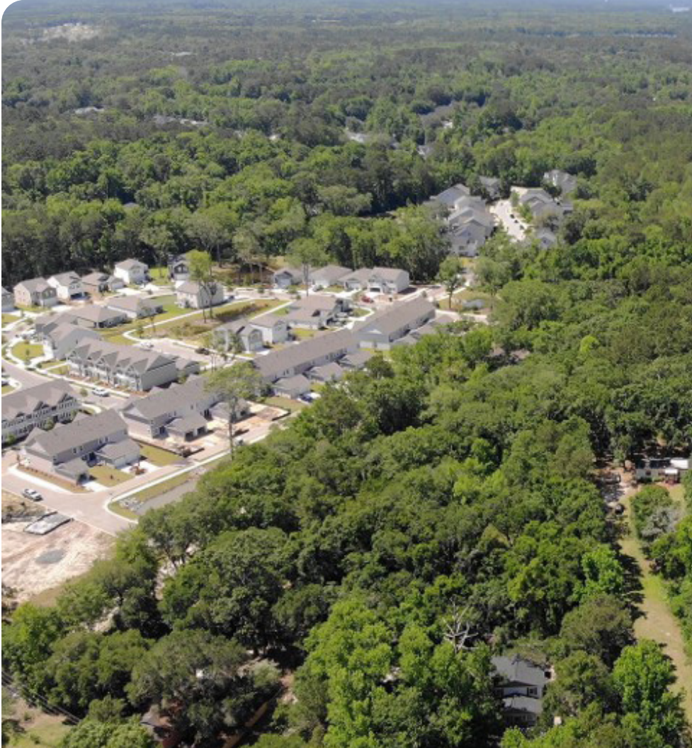
An aerial image of the Barberry Woods neighborhood on Johns Island, SC. WK Dickson's design rerouted water through the central tree-covered area to reduce flooding in the neighborhood. (Photo by WK Dickson)
