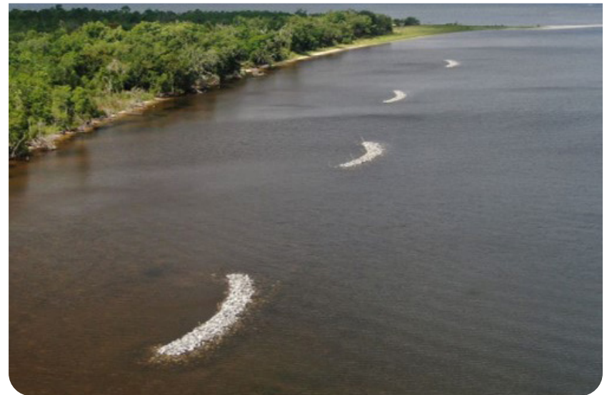
A few of the built oyster reefs that Jacobs designed for Pensacola East Bay, Florida. Top photo by NFWFMD and bottom photo by Russell C. Mick.
