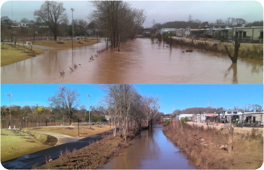
Top image: During rain event and high flood levels, Unity Park is designed to store flood waters. Bottom image: Flood levels receding after 24 hours, allowing visitors to enjoy the park.
