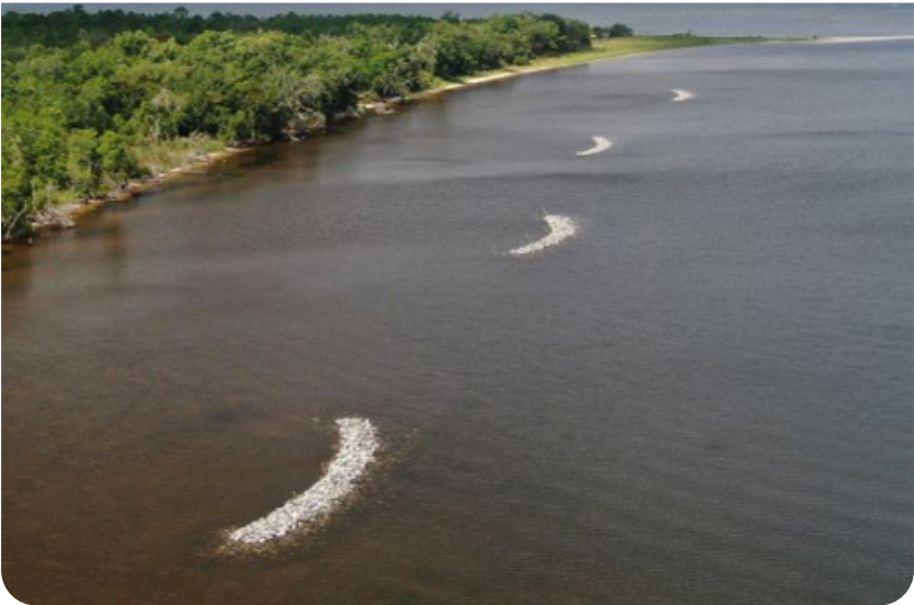
A few of the built oyster reefs that Jacobs designed for Pensacola East Bay, Florida. Top photo by NFWMD and bottom photo by Russell C. Mick.
