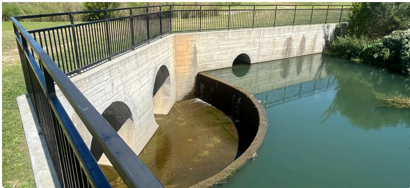
Photos are credited to Robinson Design Engineers
