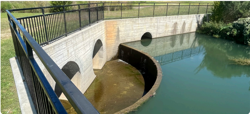
Photos are credited to Robinson Design Engineers
