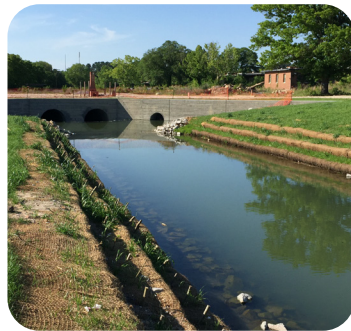
(Above) Daylighting and stream restoration of Smith Branch in Columbia, South Carolina. Of the nearly 3,000 linear feet of stream located at the park, 2,000 had been piped underground since the 1950's. RDE's stream daylighting design restored the stream to the open air and revitalized the floodplain, now a key attraction of the public park.
